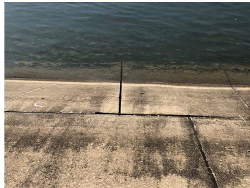
Fig. 20 Lining plate in the 9+320
