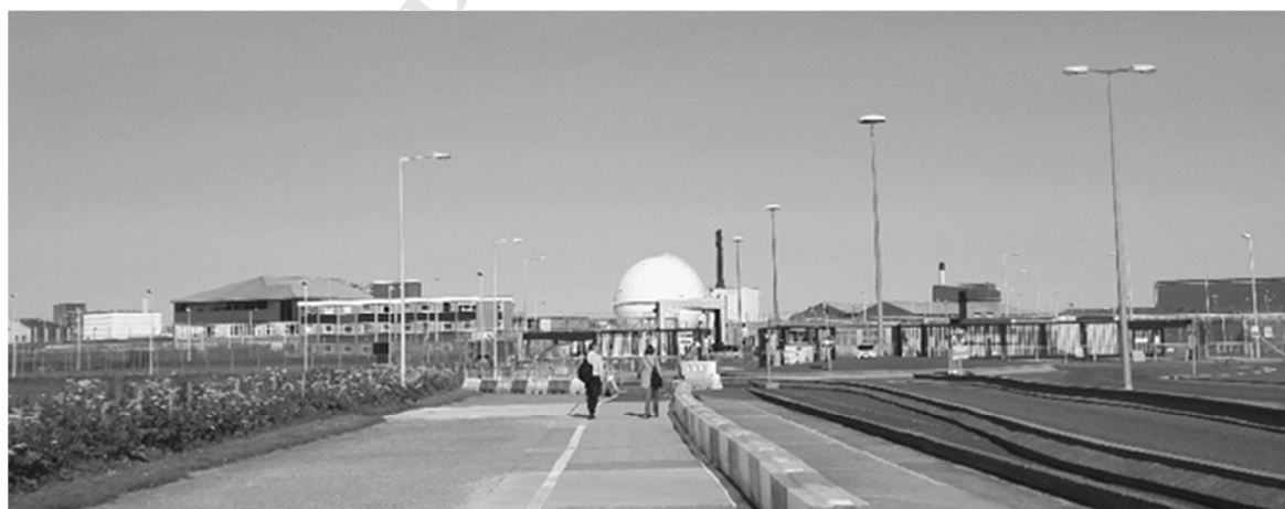
Figure 4. View of entrance to Dounreay site with the iconic 'Sphere' housing the decommissioned reactor, (Source: researcher's own, July 2017)
