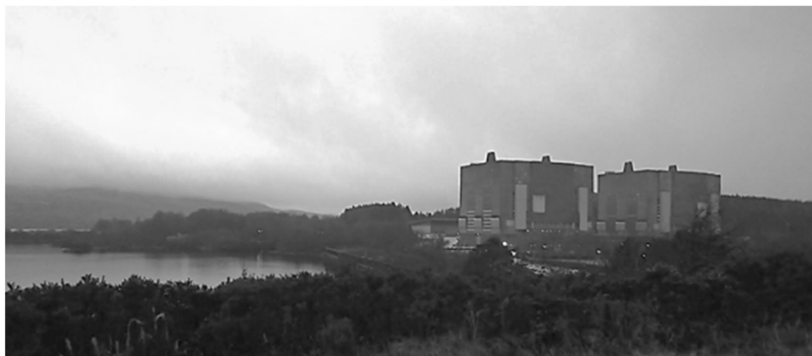
Figure 5. View of Trawsfynydd 'cathedral like' reactor buildings from viewing platform next to site (Source: researcher's own, December 2017)
