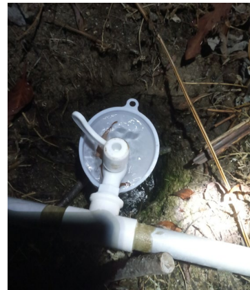
Photograph 6: Water watchers add leaching agent into networks of pipes. Chipwe/Pangwa, 2023.
