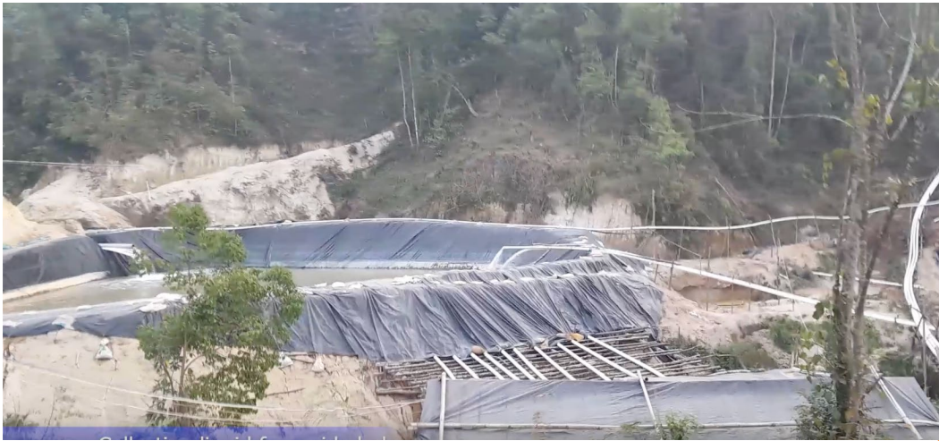
Photograph 8: Construction of collection tanks. Chipwe/Pangwa, 2023.
