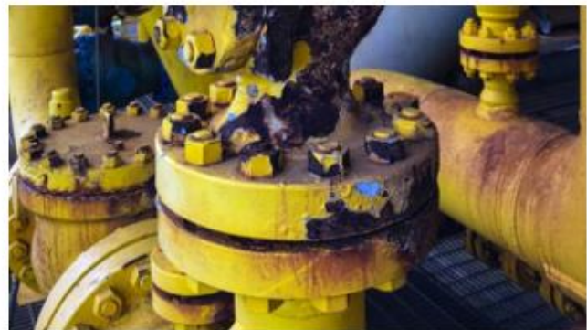
Figure 8: Crevice Corrosion (38)
