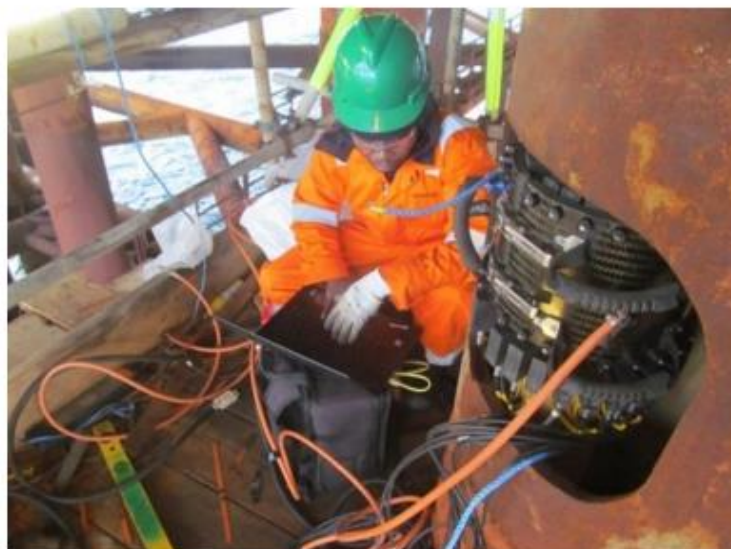
Figure 27: 6 inches gas lift riser (Long range ultrasonic testing inspection)
