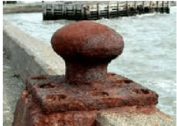
Figure 4: Uniform corrosion (21)
