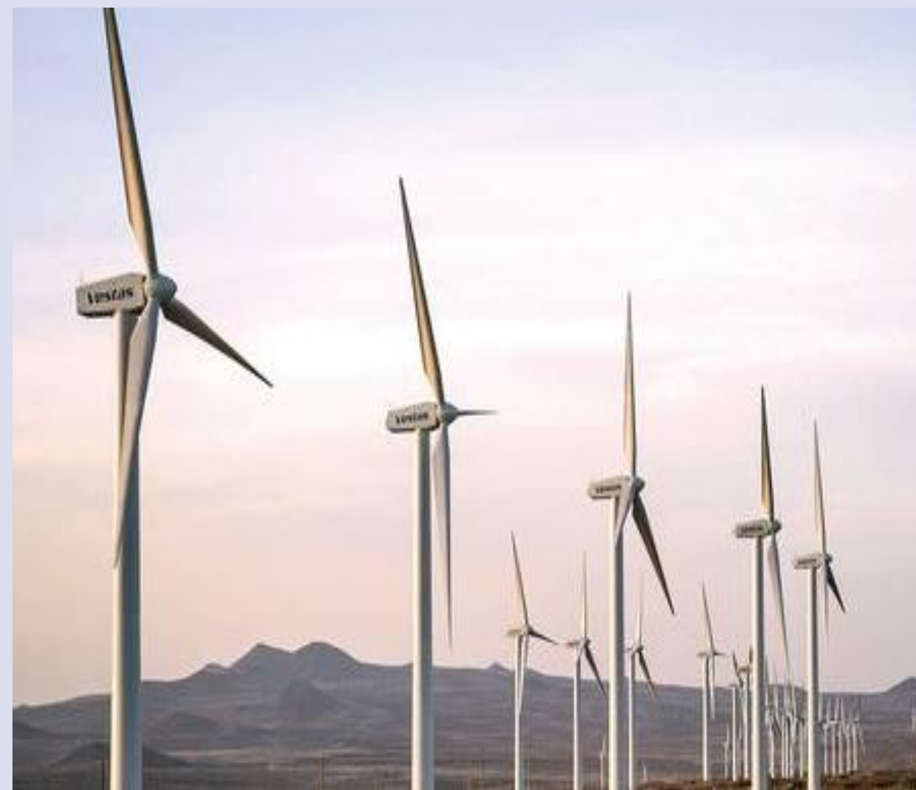
Lake Turkana wind-farm, Turkana County, Kenya © https://itwp.co.ke/
