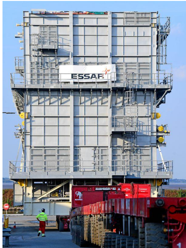
Figure 45. A ten-story hydrogen ready furnace being transported to the crude distillation unit at the Essar Refinery ((Chester and Cheshire News, 14 August 2022; https://www.cheshire-live.co.uk/news/chester-cheshire-news/giant-hydrogen-furnace-makes-way-24752714 )
