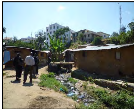
Photo 2 Open drains in Tudor, Mombasa
