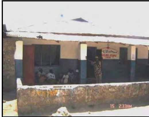
Photo 5 Protection of a local business against floods using a wall in Mombasa
