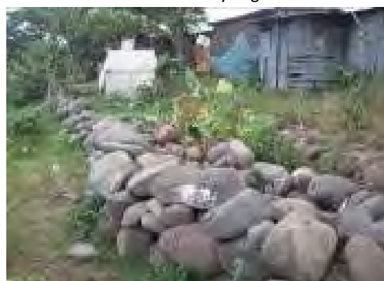
Photo 8 Contention walls built by residents in the lower part of 29 de Octubre to protect against flooding
