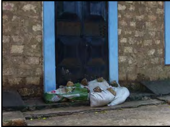
Photo 6 Protection of a house against floods using sandbags in Mombasa
