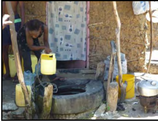
Photo 7 Protection of a community well in Tudor, Mombasa
