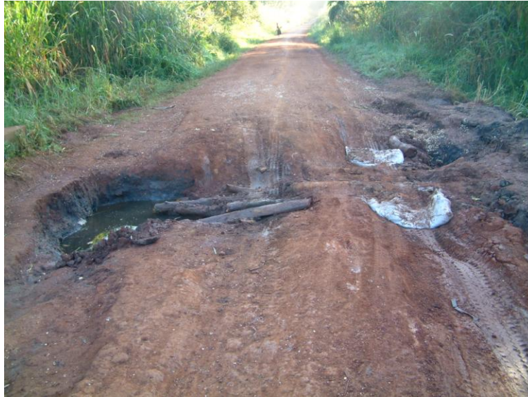
Figure 3.9: Local road conditions in Bugangaizi
