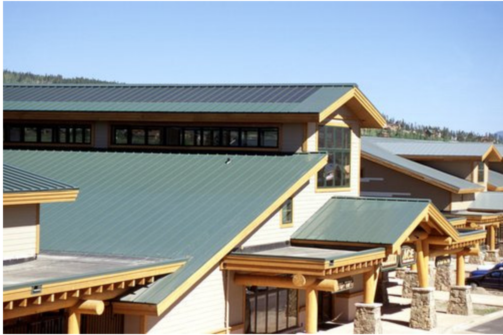
Figure 4.6: Photograph of BigHorn Home Improvement Centre [89]
