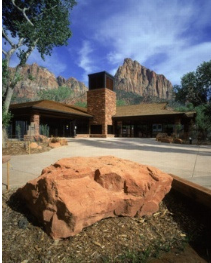
Figure 4.12: Photograph of Zion National Park Visitor's Centre [94]
