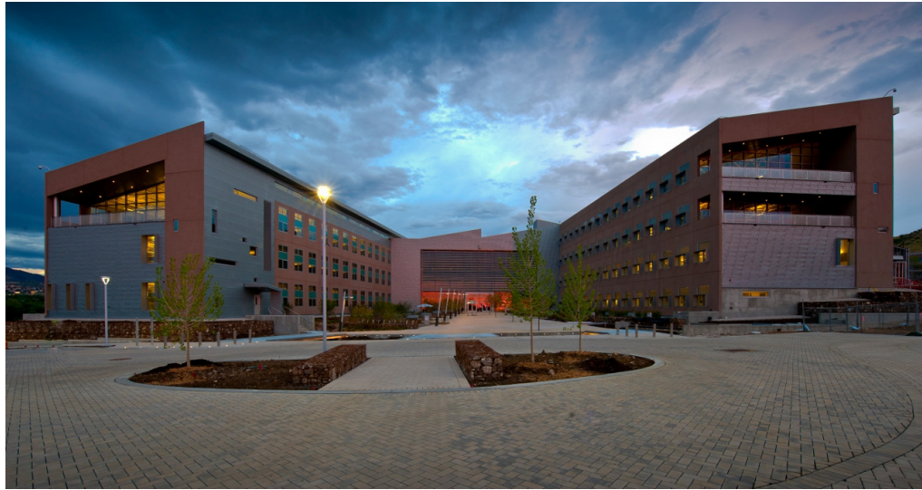
Figure 4.2: Photograph of NREL Research Support Facility [84]
