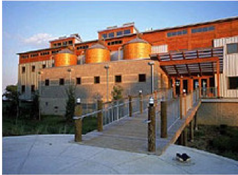
Figure 4.7: Photograph of the Chesapeake Bay Foundation's Philip Merrill Centre [90]
