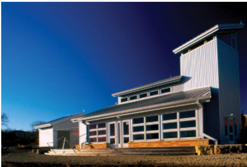
Figure 4.3: Photograph of The Science House in Minnesota [87]
