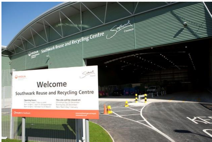
Figure 41 Southwark reuse and recycling centre
