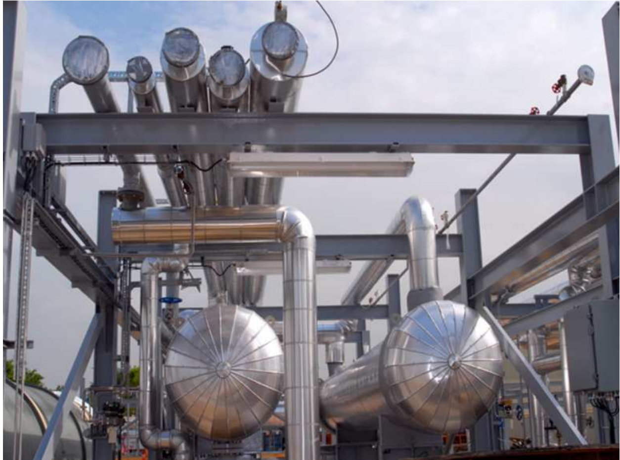
Figure 1: A shipping container-sized module consisting of two heat exchangers. The top of the module serves as a pipe rack. Photo used from permission from Mr. Bill Stanley.
