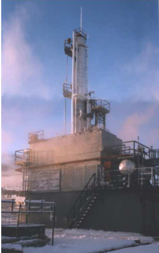
Figure 4: Modularized distillation system with heated insulated enclosure designed for low-temperature ( -150^{\circ}\text{F} , 172\text{ K} ) service (Compare with system in Figure 3, which was designed for service in ambient conditions up to 150^{\circ}\text{F} , 339\text{ K} ). Image used with permission from Mr. Bill Stanley. Image obtained by merging two separate photographs and adjusting contrast. These edits do not alter the representation of the physical system).
