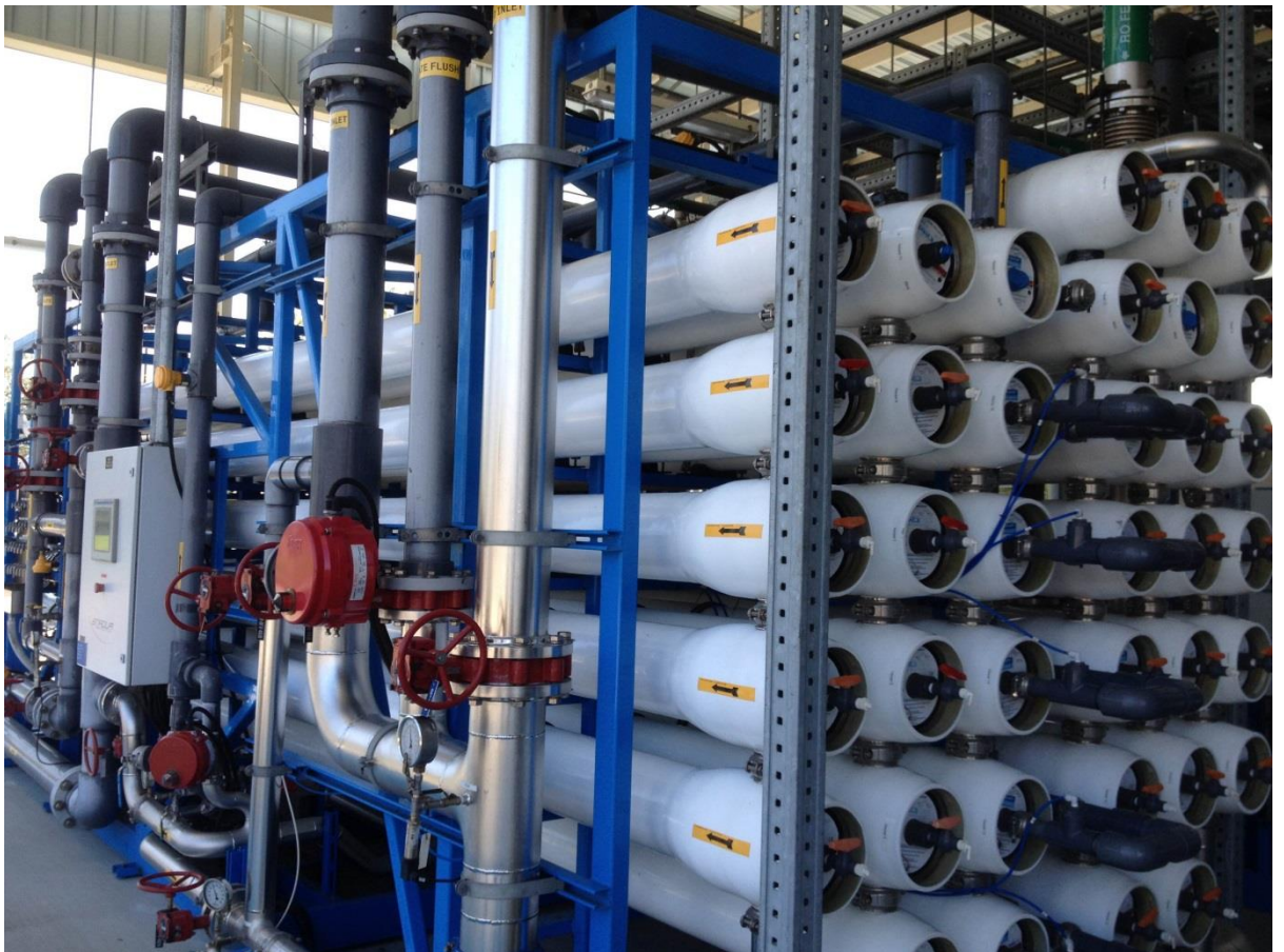
Image 1.2: Spiral-wound RO module at the North City Pure Water test facility, San Diego. Source: Joe Williams (2015)
