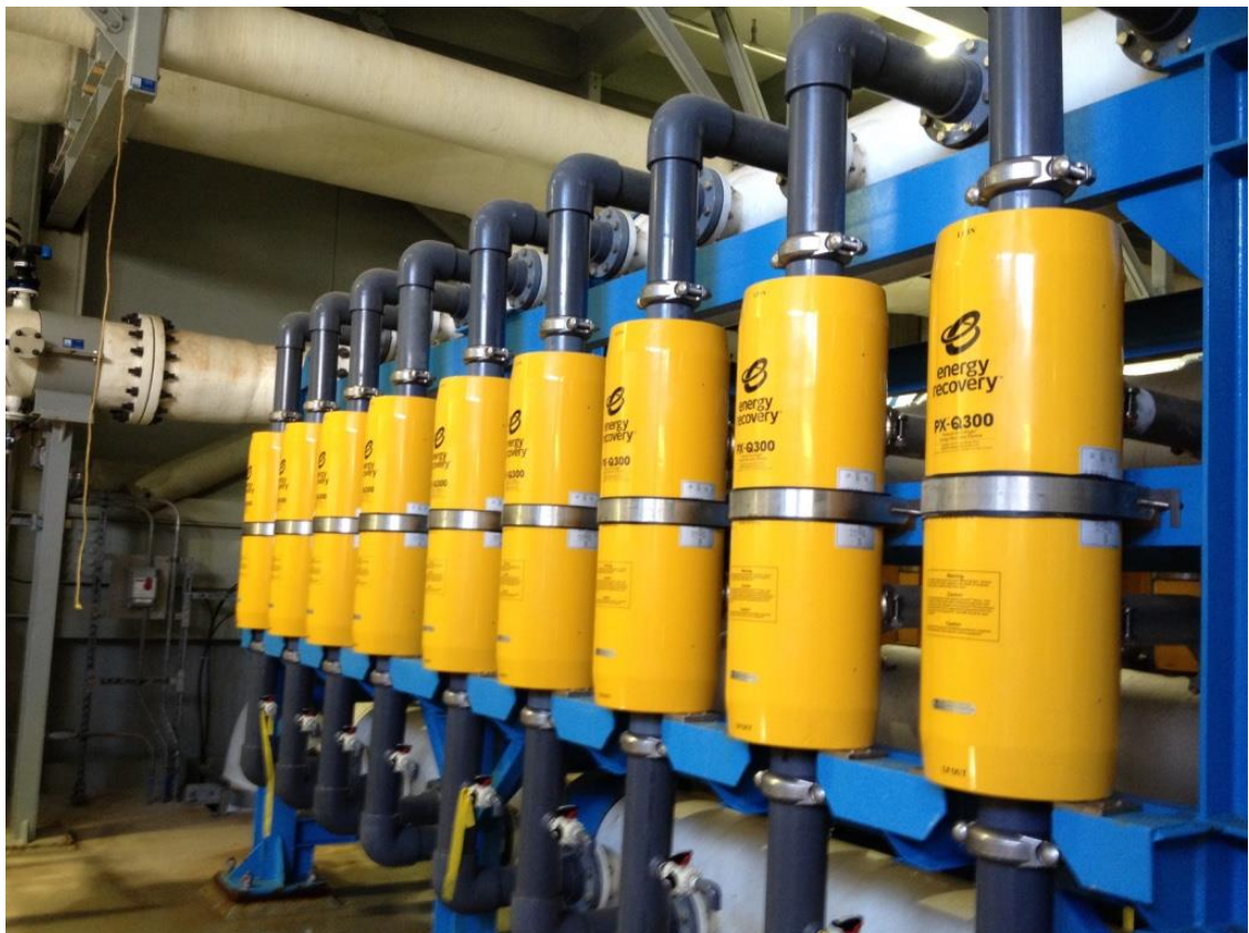
Image 6.1: Energy recovery devices reduce energy consumption at the Carlsbad Desalination Plant by 45%. Source: Joe Williams (2015)
